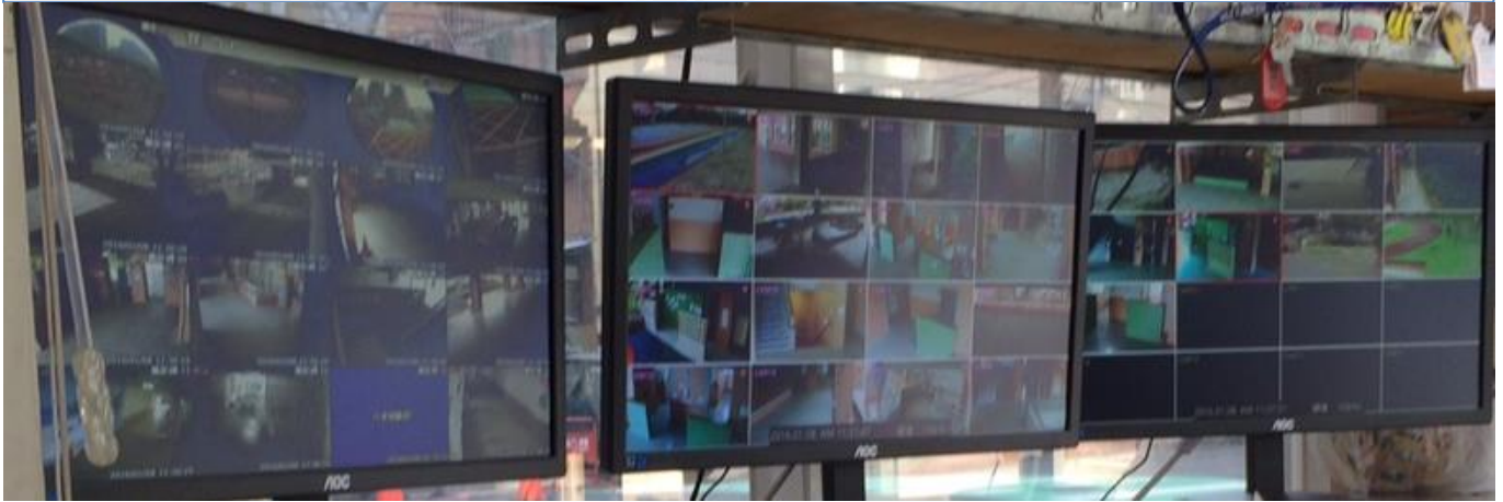
Figure 1. Because the installation is performed area by area, there is a chance to compare the old CCTV and new DTV systems side by side at the control center. The improvement is obvious. Left: CCTV analog SD system. Middle/Right: DTV full-HD system.
